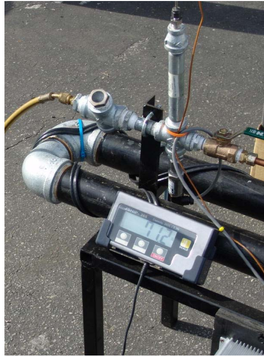
Figure 4: (a) Sight glass and instruments at inlet; (b) Cylinder scale display
