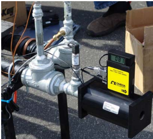
Figure 5: Flow, temperature, & pressure sensors mounted at expansion pipe outlet
